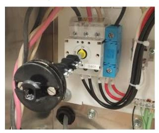
To turn on the machine, turn the black dial indicated in the figure at left clockwise so that the yellow arrow points to "on" as shown.
