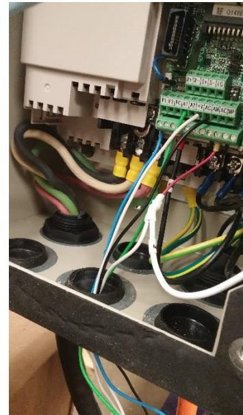
Figure 6.9 A completed rewiring of the VFD interior
